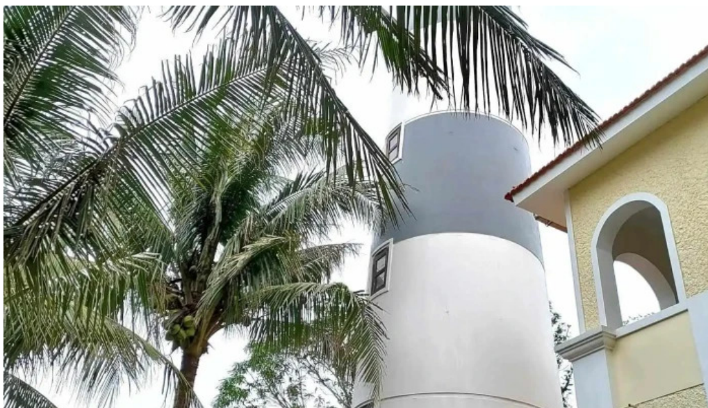
Tram hai dang cua dai cua dai lighthouse tat ca
